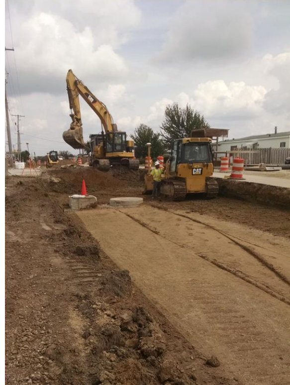
Cutting grade for the new pavement on Kossuth
