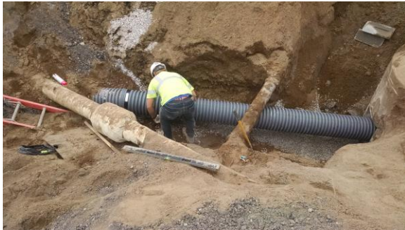
Working around lots of existing utilities underground.
