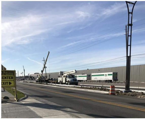
Working on the delicate operation to stand the decorative light poles
